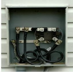
Step 2a Hi-Lug Ground Installation
