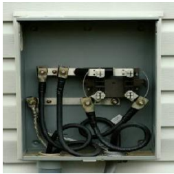
Step 2a Hi-Lug Ground Installation
